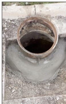
This sewer is one of fifty seven that were rebuilt therefore making storm water drain more effectively without washing away the street.
