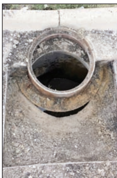
This sewer is one of fifty seven that were rebuilt therefore making storm water drain more effectively without washing away the street.
