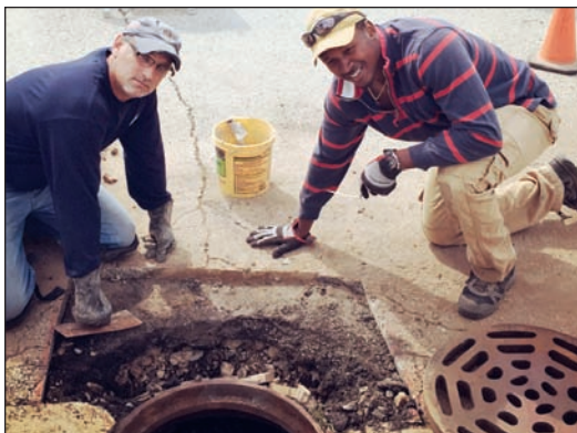
Sewer Crew - Mike Hanley and Jarvis Franklin
